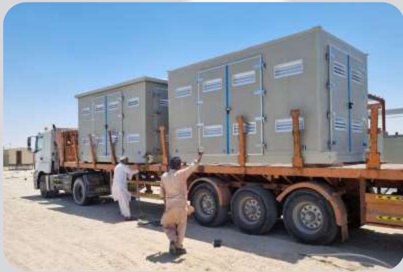
22 KV GRP PACKAGE UNIT
